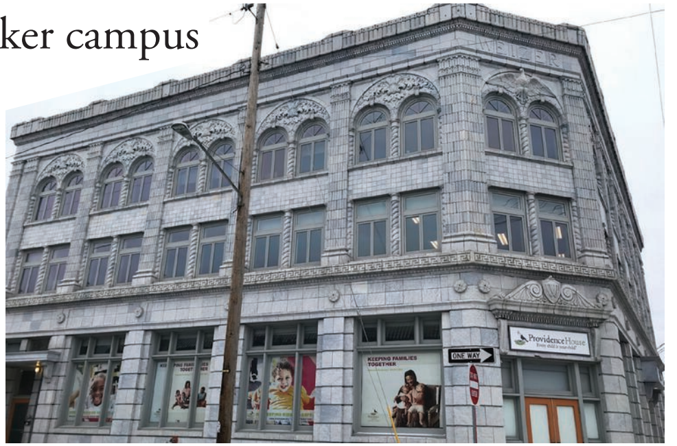
Providence House renovated the vacant Weizer building on Buckeye Road for its new East Side campus, called Hope's House. Photo by Chris Ball
